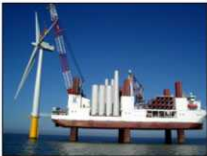
Jack-up barges cost 60M
