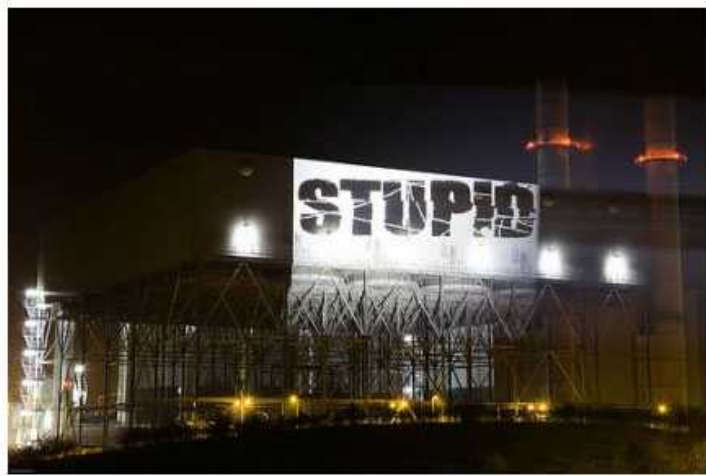
Kingsnorth Coal Power Station is definitely Stupid
